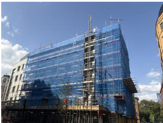
A photo of the Scaffold erection complete
