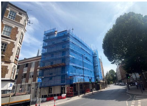
A photo of the Scaffold erection complete
