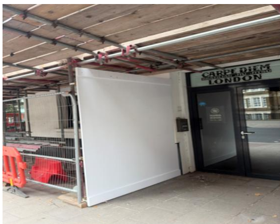
A photo of the protective gantry and hoarding surrounding the building entrance, ensuring residents can enter and exit safely while construction works take place above.
